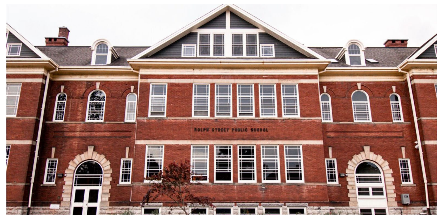
Oxford Estates in Tillsonburg: Recipient of the Paul Oberman Award for Adaptive Reuse in 2021, for transforming the former Rolph Street Public School into residential apartments
